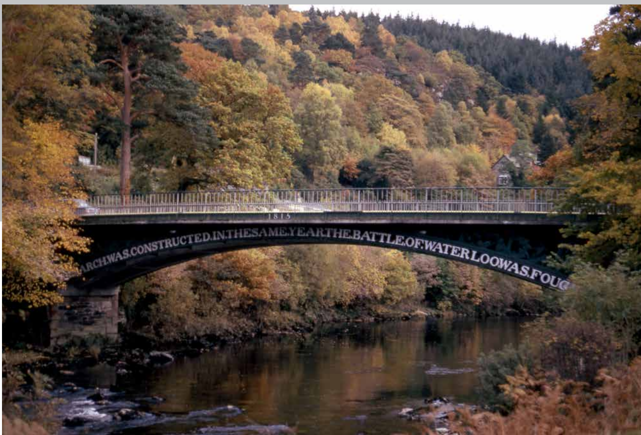
Waterloo Bridge , Betws-y-Coed, 1815. Design: Thomas Telford. Foto: Forfatteren.
